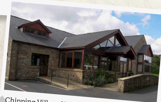
Chipping Village Hall
