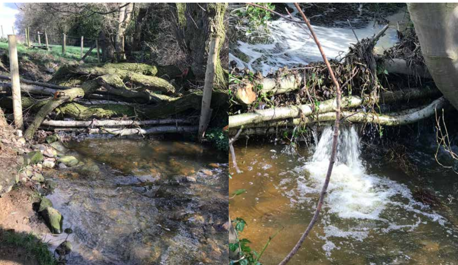
One of the newly installed leaky dams on Whitley Beck © Lune Rivers Trust
