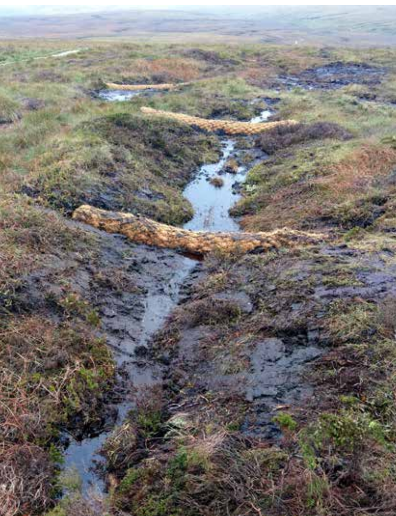
Coir rolls and reprofiling on Pendle Hill © Conservefor
