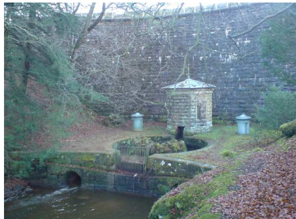
Figure 3 Lower outlet from dam
