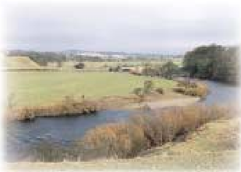
The Lune sweeps beneath Loyn Bridge
