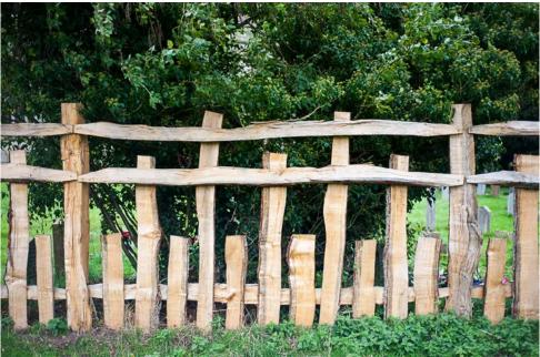
Figure 5: New deer-park fencing made by cleaving oak at Charlecote Park in Warwickshire showing pales of three heights supported by three rails. The tallest posts are 6 ft. (1.83 m) high. The fence is not set on a bank and ditch system. Photographs by the author.
