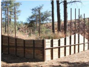
Figure 14: 'Jump-outs' in the US designed to enable large mammals such as deer/elk trapped on the highway to escape and not return: (left) a ramp on the highway side up to a drop; (right) a wooden revetment with wire supported by poles directing trapped animals from the highway at the top, to the one-way drop, and thereafter to cross the highway via an underpass. Photographs courtesy of the Arizona Game and Fish Department.
