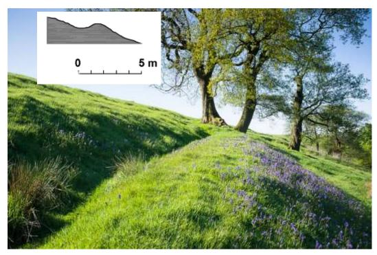
Figure 5: Eroded ditch and bank of a pale system in Leagram park, near Chipping. The park is on the left, the forest to the right. This section was probably constructed in the 1420s when the park was enlarged. The ditch was originally 8 ft. wide and 4 ft. deep. Inset courtesy of English Heritage, based on a survey by AONB volunteers.
