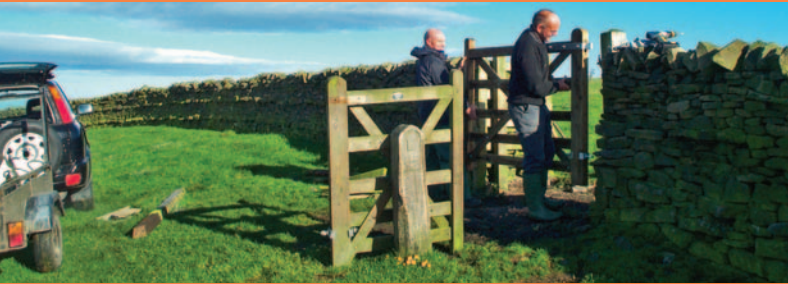
Installing a gate on a Trampler trail at Cobble Hey
