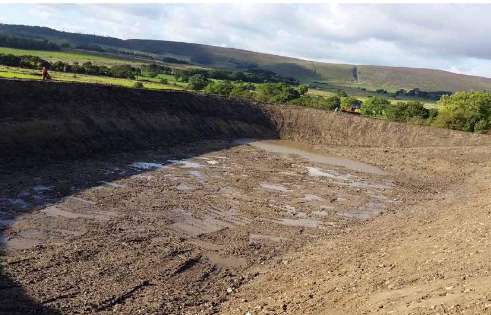
New earth bank slurry lagoon © John Stalker, Environment Agency
